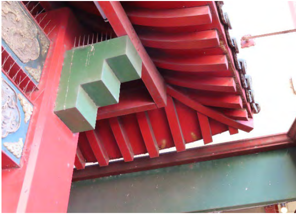
Figure 4.45 Timber bracket on the inner concrete column.
